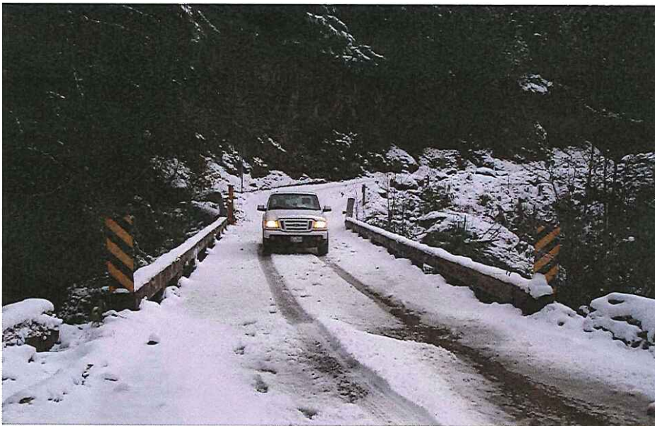
CK-2023Approach Right Bank
