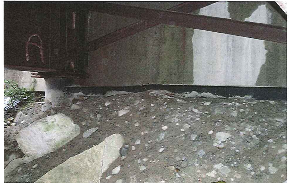
CK-2023Abutment Left Bank
