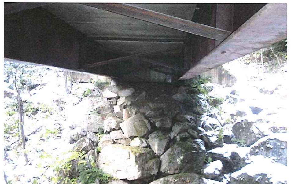
CK-2023Abutment Right Bank
